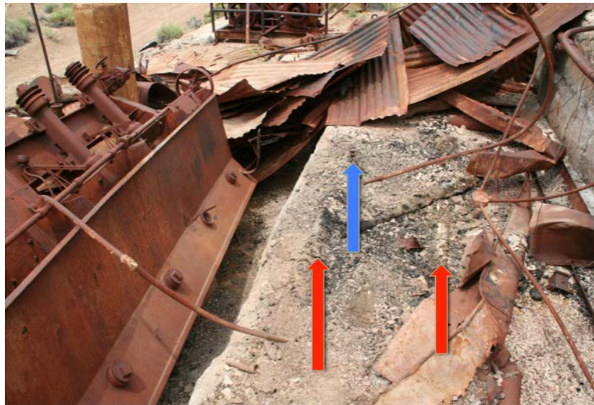
Figure 10. Roof/wall panels removed; shows the exposed elevated concrete terrace the flotation machine was originally mounted on. The red arrows indicate the location of the fire-damaged remains of heavy timber skids the machine was mounted on. The blue arrow reveals one concrete lag bolt used to secure the skids to the concrete floor.
