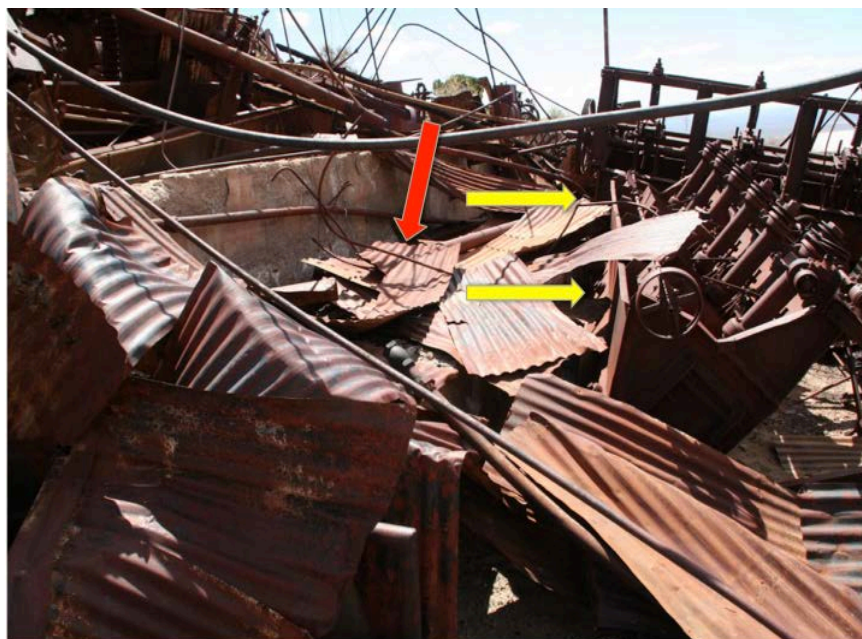
Figure 8. Red arrow points to an elevated concrete terrace covered by roof/wall panels approximately 3' off the main milling floor. Yellow arrows represent direction of travel, as flotation machine was dislocated from its normal location.
