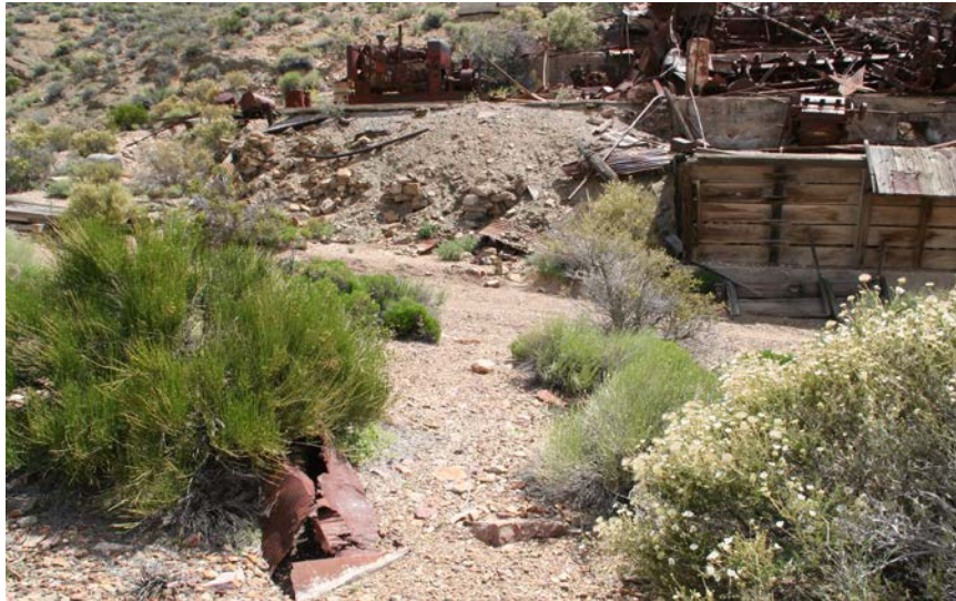
Figure 5. A roof/wall panel exhibiting effects of low-order explosive damage. This panel is located due west and approximately 90' from the Mill Building.
