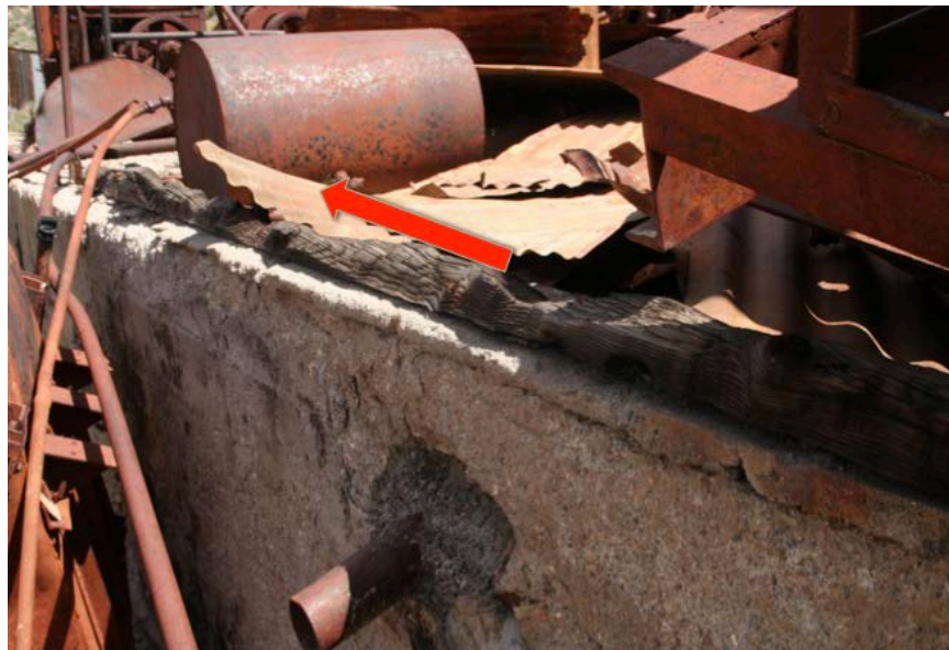
Figure 31. Red arrow points north and indicates increasing destruction to frame base plate from south to north indicating greater exposure to fire on the northerly side (northwest corner of machine room, lower tier of Mill Building).
