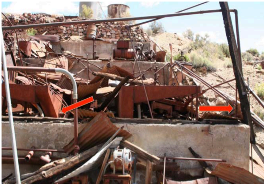
Figure 33. Demonstrates the southwest corner of the Mill Building. Construction members suffered less exposure to fire away from the flotation machine terrace and identified impact point.
