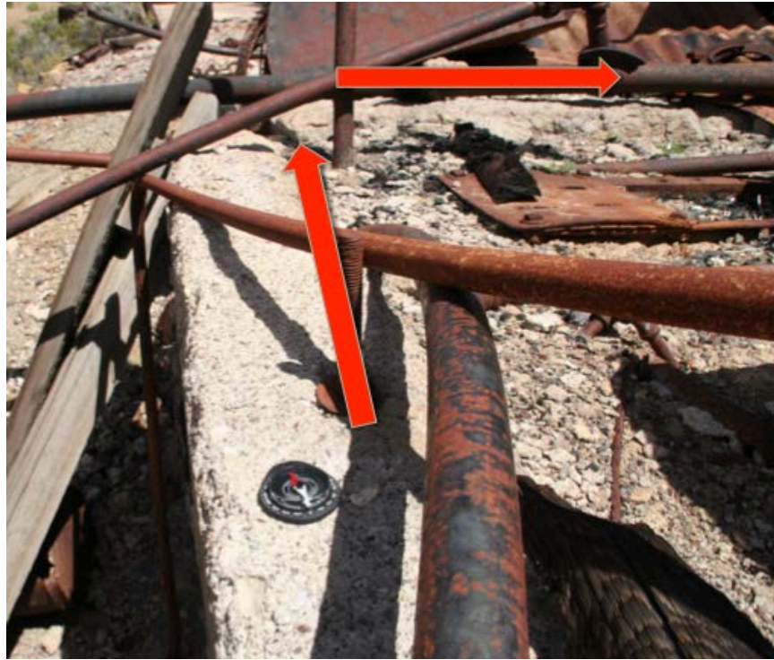
Figure 30. Northwest corner of the Mill Building lower tier wall. No remaining base plates due to consumption by fire.
