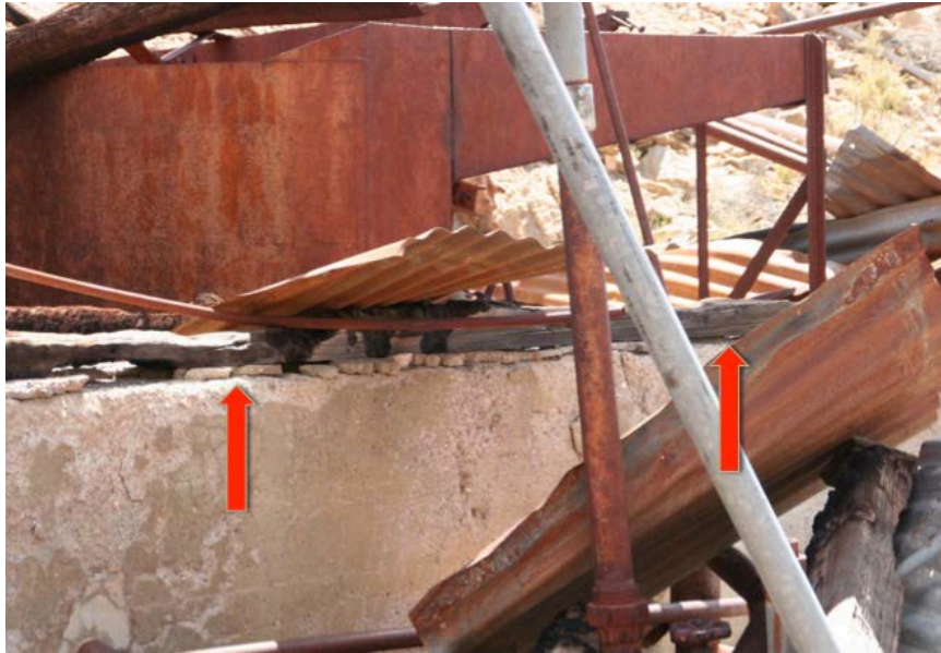
Figure 32. The remains of the frame base plate near the southwest corner of the Mill Building. This location is essentially diagonal from the flotation machine terrace and identified impact point. This photo demonstrates a reduced level of damage to construction members indicating it is away from the area of origin.
