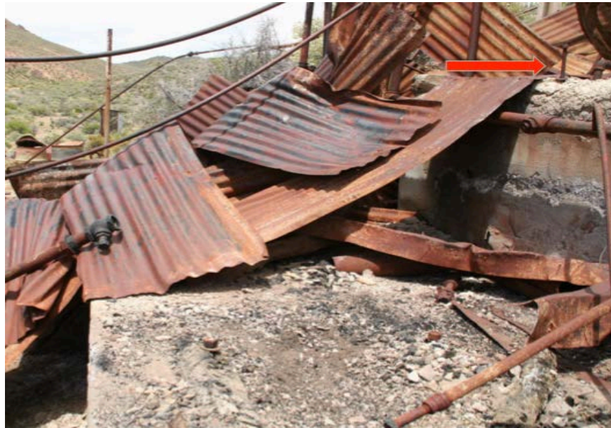
Figure 28. Red arrow indicates one lag bolt used to secure frame base plates to the retaining wall. Base plate is completely consumed by fire.
